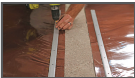
Onto a Perimeter Footing at Impediments: Seal Drago Wrap to concrete with Drago Mastic.
