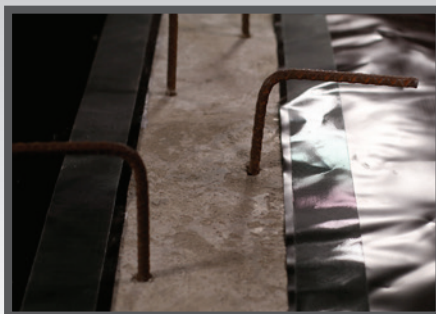
At Interior Grade Beam Impediments: Install Pango Claw onto the terminating edge of Pango Wrap.
