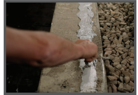
At a Location Designated by the Design Team: Seal Pango Wrap to concrete with Pango Bond and Pango Term Bar.
