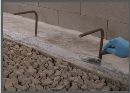
Onto a Perimeter Footing at Impediments: Seal Pango Wrap to concrete with Pango Bond and Pango Term Bar.
