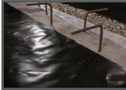
Onto Interior Grade Beams at Impediments: Seal Pango Wrap to concrete with Pango Bond and Pango Term Bar.
