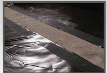
At a Location Designated by the Design Team: Install Pango Claw onto the terminating edge of Pango Wrap.
