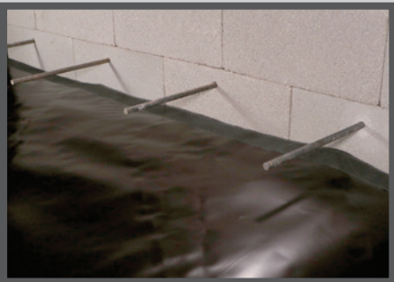
At a Foundation Wall: Install Pango Claw onto the terminating edge of Pango Wrap.
