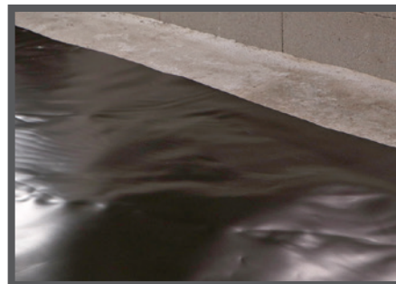
Note: The distance to which the termite/vapor barrier is extended adjacent to, onto, or completely over a footing or grade beam should be determined by the project design team.
