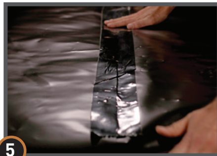
2 Unless otherwise indicated by the design professional(s) of record, unfold Pango Wrap to completely cover the placement area.
