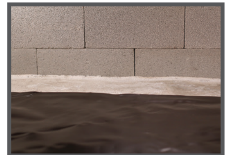
Note: The distance to which the termite/vapor barrier is extended adjacent to, onto, or completely over a footing or grade beam should be determined by the project design team.
