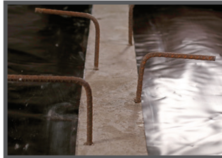
Note: Impediments may include rebar, dowels, water stops, etc. and may be located at interior grade beams in addition to perimeter walls and footings.
