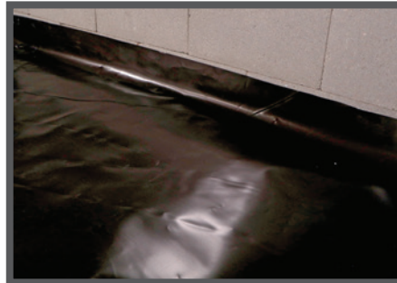
Note: Turn Pango Wrap up foundation walls or forms.
