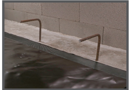
Note: Impediments may include rebar, dowels, water stops, etc. and may be located at interior grade beams in addition to perimeter walls and footings.
