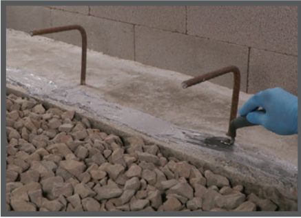
Onto a Perimeter Footing at Impediments: Seal Pango Wrap to concrete with Pango Bond and Pango Term Bar.
