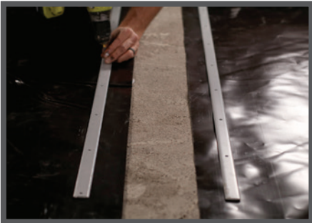
Utilize Pango Term Bar to fasten Pango Wrap to concrete or masonry.
