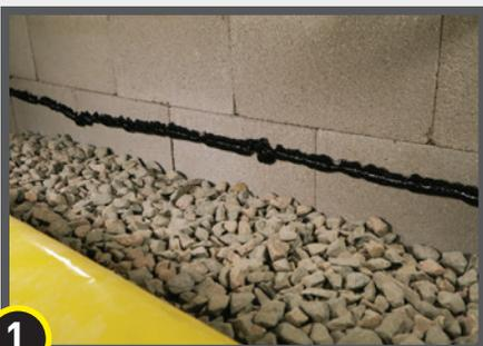
**1** Apply Stego Mastic to the foundation wall at the anticipated edge of the subsequently applied Stego Wrap at the height of the slab or impediments.
