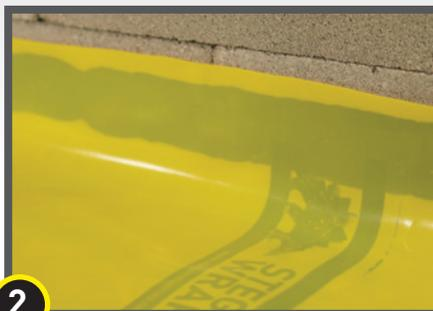
**2** Press Stego Wrap firmly against the applied Stego Mastic on the foundation wall.
