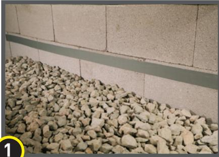
**1** Remove the release liner on one side of StegoTack Tape and stick to foundation wall at the height of the slab or at impediments.
