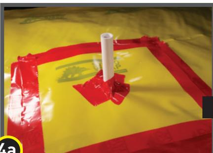
**4a** Seal around the base of the pipe using Stego Tape. **OR...**
