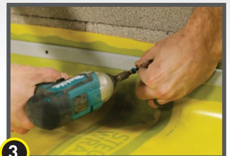
**3** If consistent, continuous pressure will not be applied (e.g. by a concrete slab), Stego Term Bar may be necessary.
