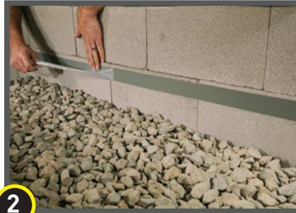
**2** When ready to apply Stego Wrap, remove the exposed release liner from StegoTack Tape.
