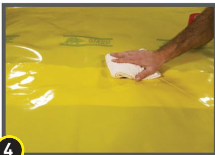
**4** Ensure Stego Wrap is clean and dry when applying Stego Tape.
