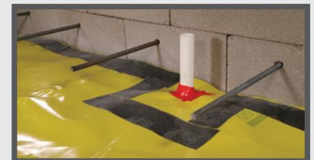
If protrusions or penetrations are determined to be impediments to applying Stego Crete Claw Tape along the perimeter terminating edges of Stego Wrap, route Stego Crete Claw Tape around the impediment, as close to the impediment as possible, and continue along the terminating edge of Stego Wrap on the opposite side of the impediment.
