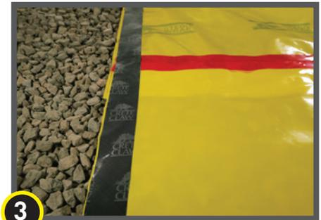
**3** Install Stego Crete Claw Tape last for a successful installation.
