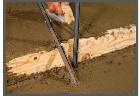
Beast Form Stake is strong enough to withstand a beating during concrete placement while holding its shape. It is easy to remove and reusable for the next job.
