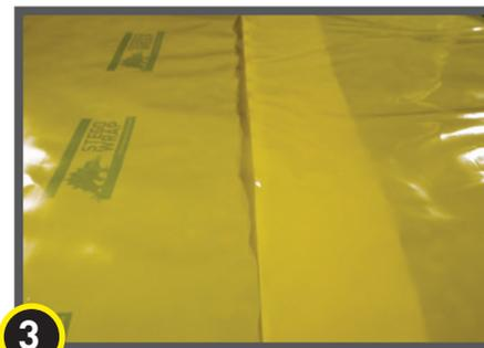
**3** All joints/seams should be overlapped a minimum of 6 inches.
