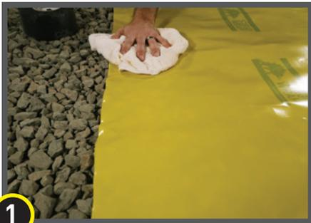
**1** Ensure Stego Wrap is clean and dry when applying Stego Crete Claw Tape.
