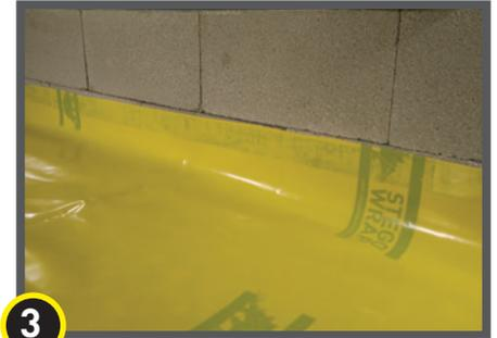
**3** Press Stego Wrap firmly against StegoTack Tape to secure.
