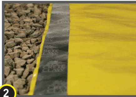
**2** Apply Stego Crete Claw Tape as close as possible to the terminating edge of Stego Wrap.
