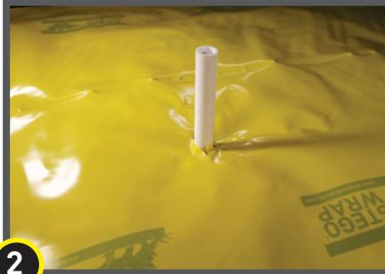
**2** Pull material over and flatten. Clean area of adhesion where Stego Tape will be applied.
