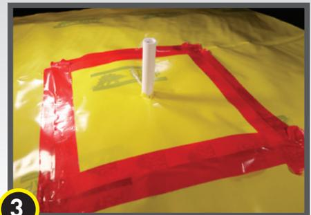
**3** Seal all sides of the pipe boot with Stego Tape.
