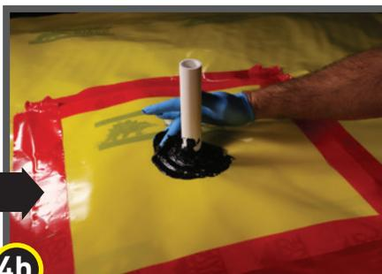
**4b** Seal around the base of the pipe with Stego Mastic. Note: apply using disposable glove, paint brush, or similar.
