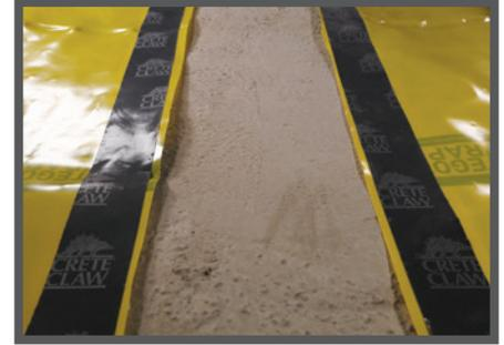
At a Location Designated by the Design Team: Install Stego Crete Claw onto the terminating edge of Stego Wrap.
