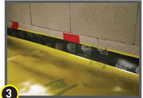
Apply the entire 3" width of Stego Crete Claw Tape on the perimeter edge of Stego Wrap.
