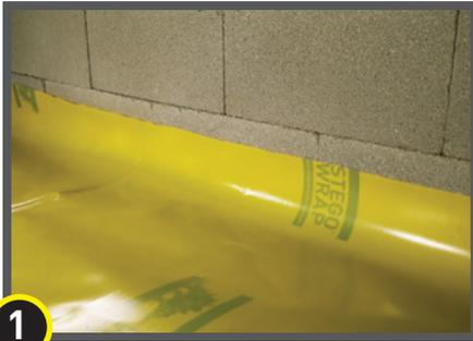
Extend Stego Wrap up the vertical surface, likely to the height of the slab.
