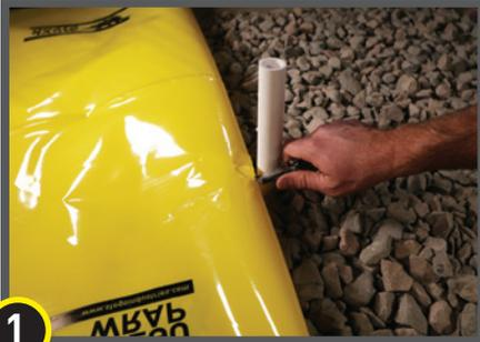
**1** Install Stego Wrap around pipe penetrations by slitting/cutting material as needed. Try to minimize the void space created.
