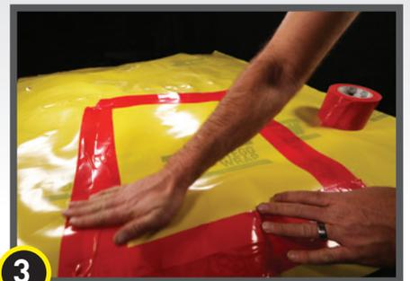
**3** Measure and cut a piece of Stego Wrap to cover damaged area 6" in all directions. Seal patch with Stego Tape.
