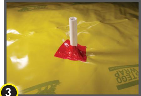
**3** If Stego Wrap is close to pipe and void space is minimized then seal around pipe penetration with Stego Tape and/or Stego Mastic.
