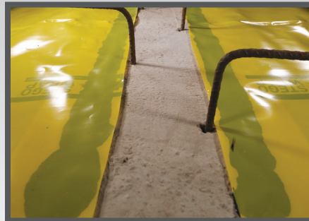
Onto Interior Grade Beams at Impediments: Seal Stego Wrap to concrete with Stego Mastic.
