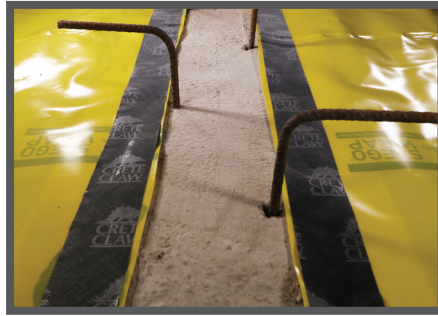
At Interior Grade Beam Impediments: Install Stego Crete Claw onto the terminating edge of Stego Wrap.
