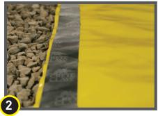
Apply Stego Crete Claw Tape as close as possible to the terminating edge of Stego Wrap.
