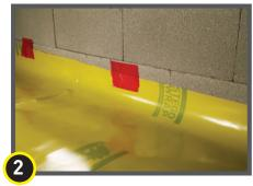
**Optional:** Temporarily secure Stego Wrap to the foundation wall with a small piece of Stego Tape.
