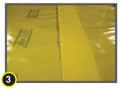
All joints/seams should be overlapped a minimum of 150 mm (6").
