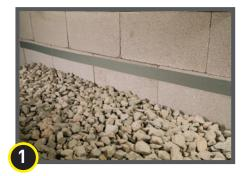
Remove the release liner on one side of StegoTack Tape and stick to foundation wall at the height of the slab or at impediments.
