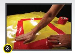
Measure and cut a piece of Stego Wrap to cover damaged area 150 mm (6") in all directions. Seal patch with Stego Tape.
