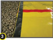
Install Stego Crete Claw Tape last for a successful installation.
