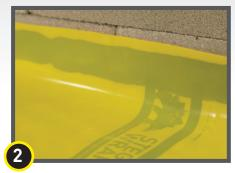
Press Stego Wrap firmly against the applied Stego Mastic on the foundation wall.
