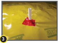
If Stego Wrap is close to pipe and void space is minimised then seal around pipe penetration with Stego Tape and/or Stego Mastic.
