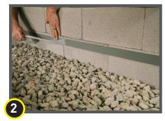
When ready to apply Stego Wrap, remove the exposed release liner from StegoTack Tape.
