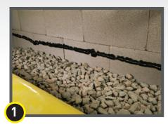
Apply Stego Mastic to the foundation wall at the anticipated edge of the subsequently applied Stego Wrap at the height of the slab or impediments.
