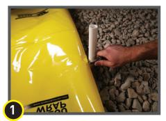
Install Stego Wrap around pipe penetrations by slitting/cutting material as needed. Try to minimise the void space created.
