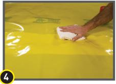
Ensure Stego Wrap is clean and dry when applying Stego Tape.
