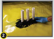
Dab Stego Mastic with disposable glove, paint brush, or similar, making sure entire void space is sealed. Note: If pipe penetrations are abutted against
