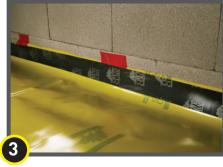
Apply the entire 75 mm (3") width of Stego Crete Claw Tape on the perimeter edge of Stego Wrap.
