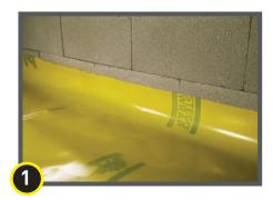
Extend Stego Wrap up the vertical surface, likely to the height of the slab. Note: See Where to Terminate the Stego Wrap, page 5.
