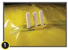
Cut a slit the size to accommodate the width of the multiple pipes. Try to minimise the void space created.
