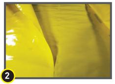
Unless otherwise indicated by the design professional(s) of record, unfold Stego Wrap to completely cover the placement area.
