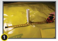
Cut a detail patch to a size and shape that creates a 150 mm (6") overlap on all edges around the void space at the base of the pipe.
