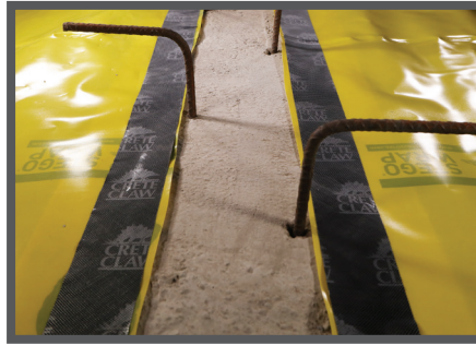
At Interior Grade Beam Impediments: Install Stego Crete Claw onto the terminating edge of Stego Wrap.
