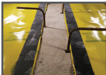
Note: Impediments may include rebar, dowels, water stops, etc.
