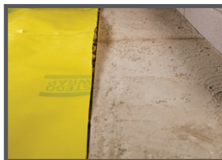
Note: The distance to which the vapour barrier is extended adjacent to, onto, or completely over a footing or grade beam should be determined by the project design team.
