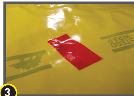
Center Stego Tape over small hole or slice in Stego Wrap.
