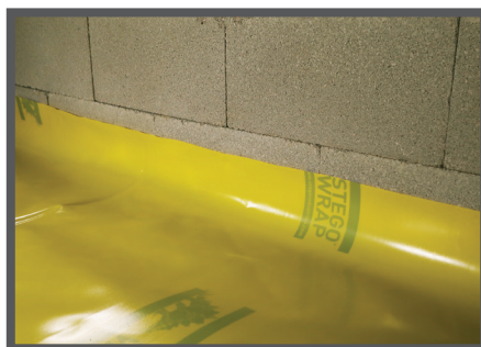
Note: Turn Stego Wrap up foundation walls or forms.
