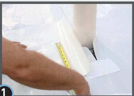
**1** Cut a detail patch/boot of StegoCrawl Wrap to a size and shape that creates a 6" overlap on all edges around the void space at the base of the penetration.
