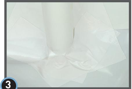
**3** Seal around the penetration using StegoCrawl Tape.
