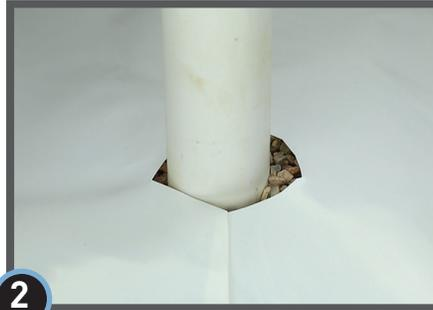
**2** Lay StegoCrawl Wrap flat around penetrations. Clean the area of adhesion where StegoCrawl Tape will be applied.
