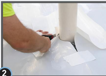
**2** A single straight cut from the edge to the center of the detail patch may be necessary for many crawl space penetrations.
