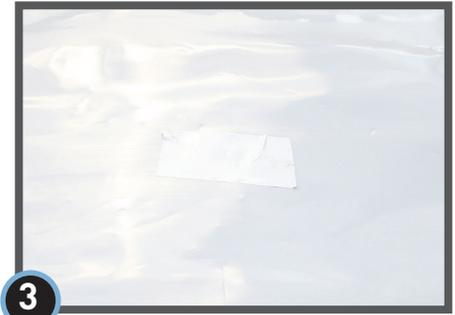
**3** Center and apply StegoCrawl Tape over small hole or slice in StegoCrawl Wrap.
