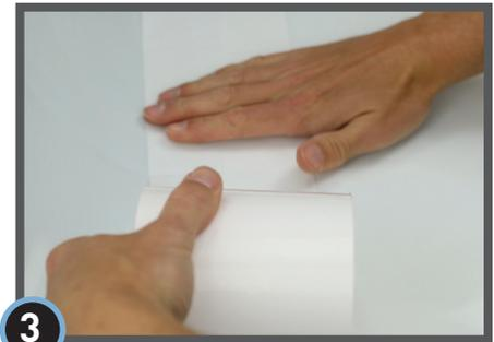
**3** Ensure StegoCrawl Wrap is clean and dry when applying StegoCrawl Tape.
