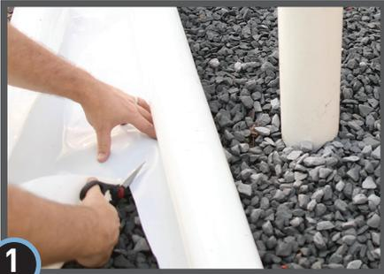
**1** Install StegoCrawl Wrap around pipe penetrations by slitting/cutting material as needed. Try to minimize the void space created.
