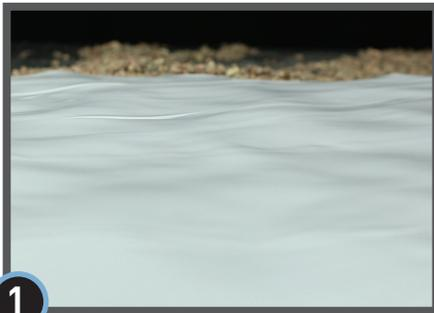
**1** Unroll (and unfold) StegoCrawl Wrap to cover entire crawl space floor area.
