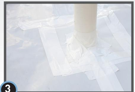
**3** Seal all sides of the patch and around the penetration with StegoCrawl Tape.
