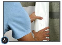
Press StegoCrawl Wrap firmly against StegoTack Tape to secure to the foundation wall.
