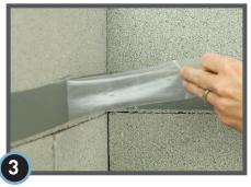
When ready to adhere StegoCrawl Wrap, remove the exposed release liner from StegoTack Tape.
