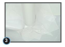
Seal around the penetration using StegoCrawl Tape.
