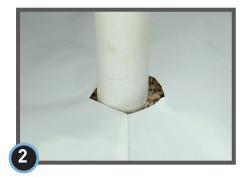
Lay StegoCrawl Wrap flat around penetrations. Clean the area of adhesion where StegoCrawl Tape will be applied.
