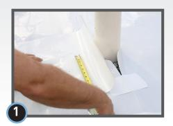
Cut a detail patch/boot of StegoCrawl Wrap to a size and shape that creates a 6" overlap on all edges around the void space at the base of the penetration.
