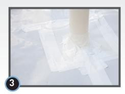
Seal all sides of the patch and around the penetration with StegoCrawl Tape.
