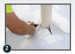
A single straight cut from the edge to the center of the detail patch may be necessary for many crawl space penetrations.
