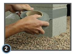
Remove the release liner on one side of StegoTack Tape and adhere to the support column. Be sure to apply firm pressure to maximize bond to the column.
