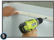
Mechanically attach StegoCrawl Term Bar, being sure to line up with the StegoTack Tape.
