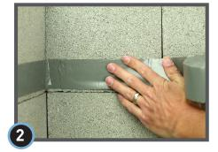
Remove the release liner on one side of StegoTack Tape and adhere to the foundation wall. Be sure to apply firm pressure to maximize bond to the wall surface.
