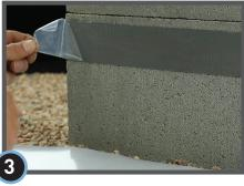
When ready to adhere StegoCrawl Wrap, remove the exposed release liner from StegoTack Tape.
