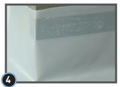
Press StegoCrawl Wrap firmly against StegoTack Tape to secure to the column.
