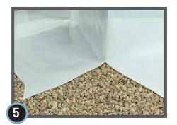
To help allow StegoCrawl Wrap to lay flat on the horizontal ground surface, relief slits can be cut into the material or detail strip.
