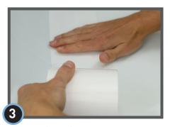
Ensure StegoCrawl Wrap is clean and dry when applying StegoCrawl Tape.
