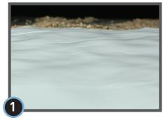
Unroll (and unfold) StegoCrawl Wrap to cover entire crawl space floor area.
