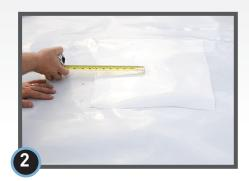
Clean area of adhesion. Measure and cut a piece of StegoCrawl Wrap to cover damaged area 6" in all directions. Then center the Stego-Crawl Wrap patch to cover the damaged area 6" in all directions.
