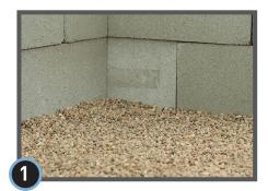
The foundation wall should be free from dirt, debris, and moisture at the point where StegoCrawl Wrap will be sealed and attached.
