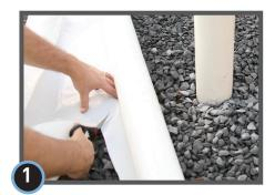
Install StegoCrawl Wrap around pipe penetrations by slitting/cutting material as needed. Try to minimize the void space created.
