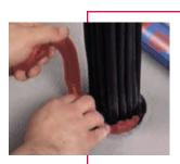
Non-hardening, intumescent putty is easily installed and removed making it the perfect choice for cable penetrations requiring occasional retrofitting.
