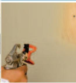
3. Apply Sto EmeraldCoat® onto the entire wall surface. Sto EmeraldCoat® can be used beneath various claddings.
