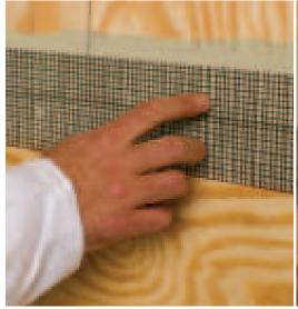
1. Apply Sto EmeraldCoat® by spray or roller liberally to all vertical and horizontal sheathing joints. Embed 4"(400 mm) StoGuard Fabric.
