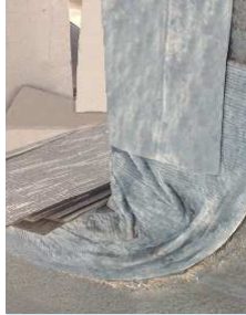
Difficult to fold and adhere at corners
