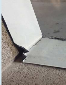
Tearing of the membrane
