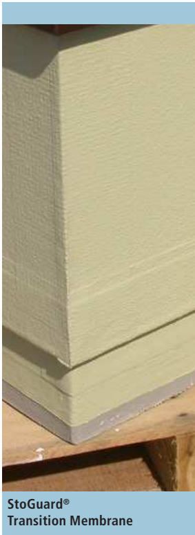
Difficult to fold and adhere at corners
