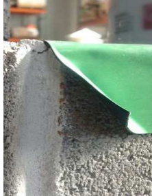
Peeling along edges
