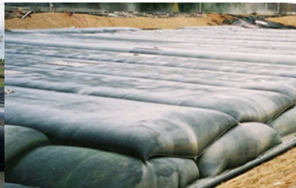
GEOTUBE ® containers in activated sludge basin at paper plant.
