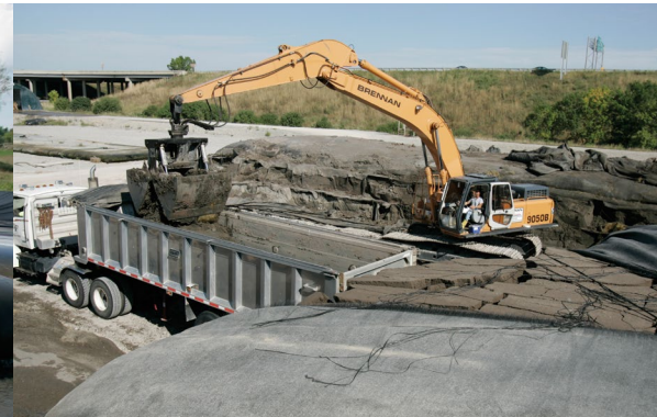
Dewatered sludge being removed from a GEOTUBE ® container with a backhoe.
