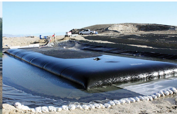
Gold mine tailings from barren and pregnant ponds dewatering in GEOTUBE ® containers.
