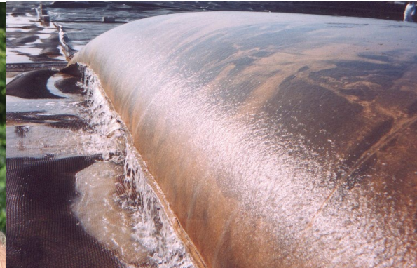
Water draining from a GEOTUBE ® container.
