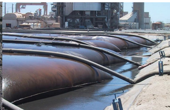
GEOTUBE ® containers at power plant being used to dewater fly ash.
