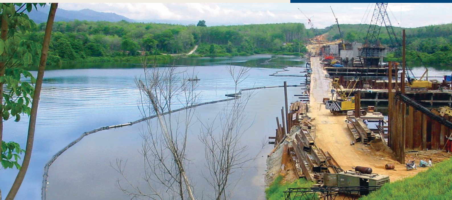
Geotube® Silt Curtain deployed to prevent the dispersion of suspended solids.
