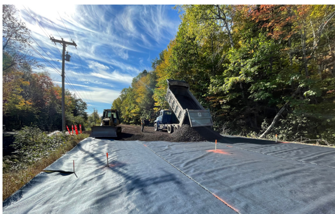
Figure 3: End dumping aggregate
