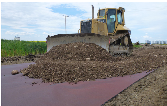
Figure 4: Spreading aggregate over geosynthetic
