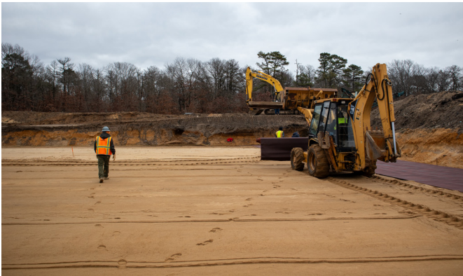
Figure 1: Subgrade preparation
