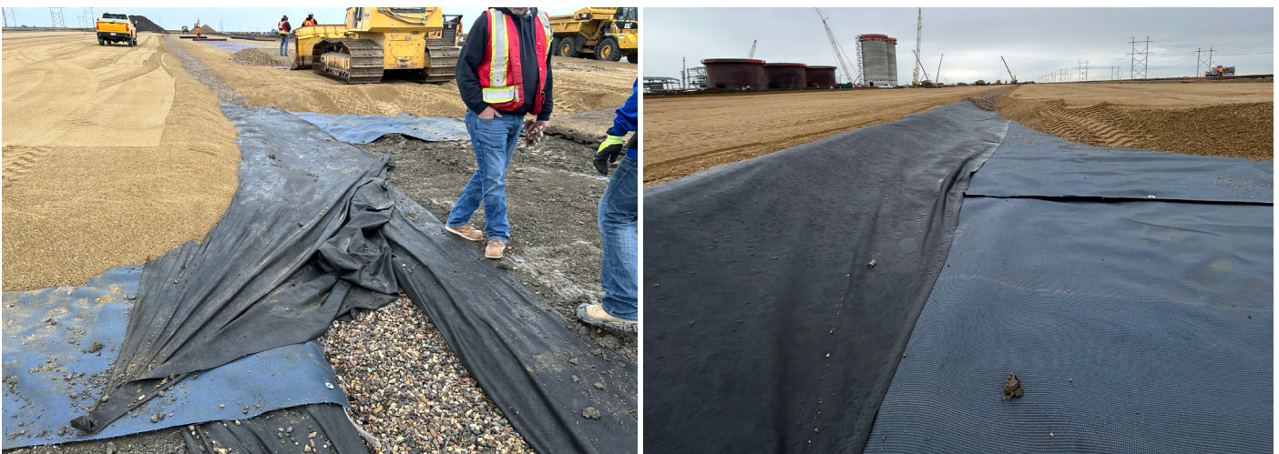
Image 12: MIRAFI H 2 Ri termination into edge drain
