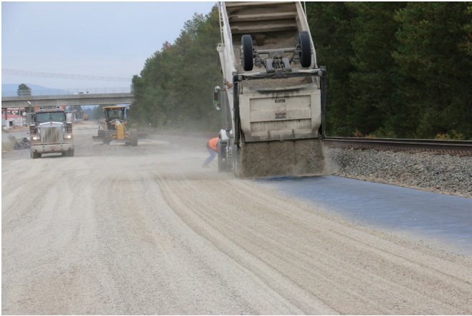
Image 17: Gate set to spread 1 in (25 mm) lift allowing a full spread over one roll
