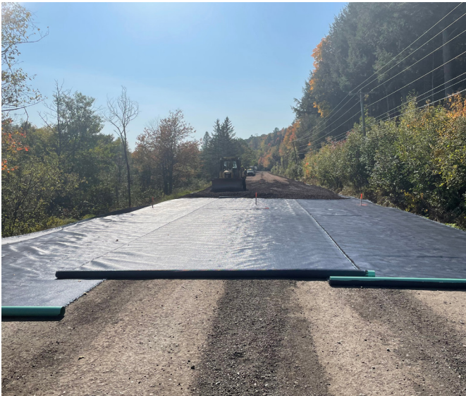
Image 3: Center roll at the high point moving water to the left and right
