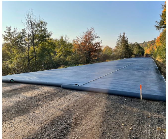
Image 4: Super elevation on left, moving water from left to right
