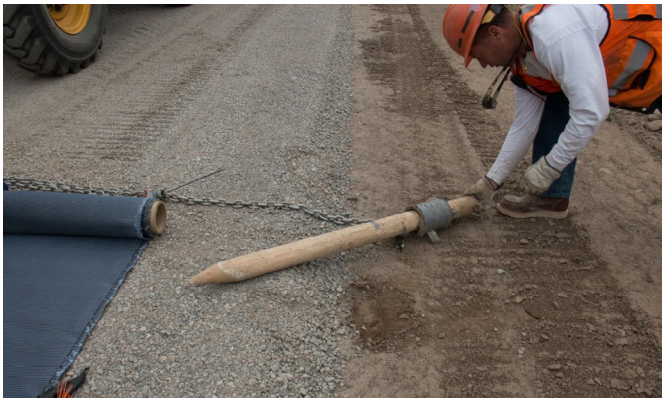
Image 14: Fence posts used as end holders for unrolling
