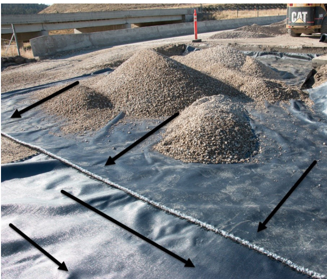
Image 5: Bridge approach, routing water away from structure
