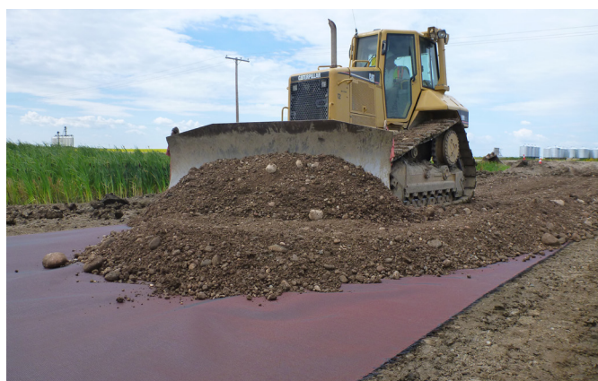
Figure 4: Spreading aggregate over geosynthetic
