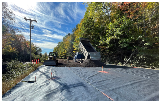
Figure 3: End dumping aggregate
