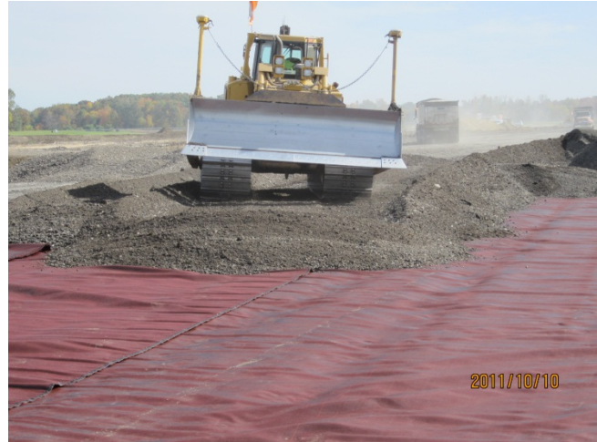
Image 4 – Spreading aggregate over geosynthetic
