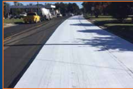
Mirafi® MPM Composite Paving Mat A fiberglass/polyester pavement interlayer designed to create a moisture-resistant barrier, retard reflective cracking and stand up to high-temperature hot-mix designs.
