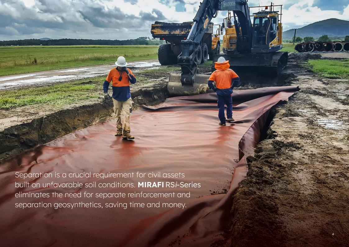
In some cases, single-layer geotextiles allowed for 15% more fines contamination of the base course than MIRAFI RS380*i* and RS580*i*.
