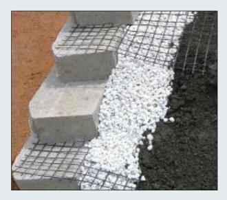
walls. It is produced with strong fibers that reinforce the entire soil structure. Other open mesh grids, such as safety fence or deer netting, are much weaker than Miragrid® 2XT geogrid and do not provide adequate reinforcement.
