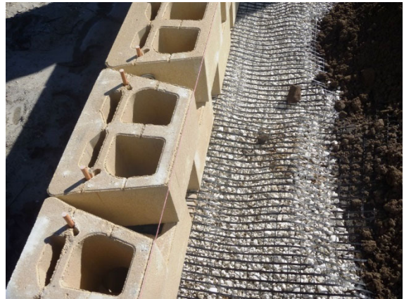
Figure 1. Miragrid® 5XT in SRW.
