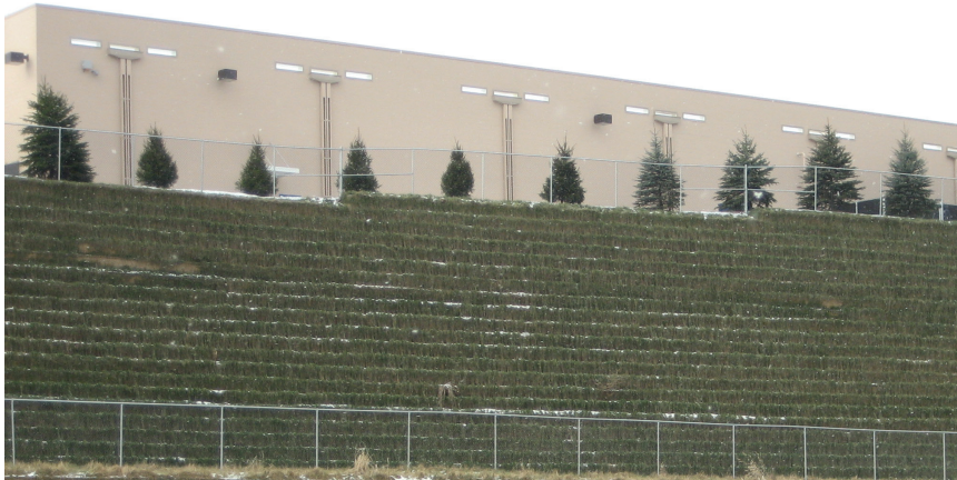
Lowe's Store, Western Hills, OH, Height = 65 1H:3V Miramesh GR inside wire basket wall.
