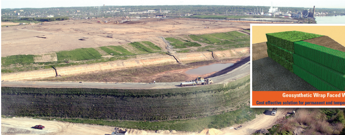
Cherry Island Landfill Expansion, Delaware River, Miramesh GR inside wire basket facing, Height = 75 ft.
