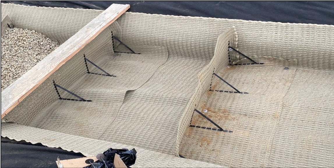
**Figure 4- Alignment and placement of baffles in bottom of excavation**
