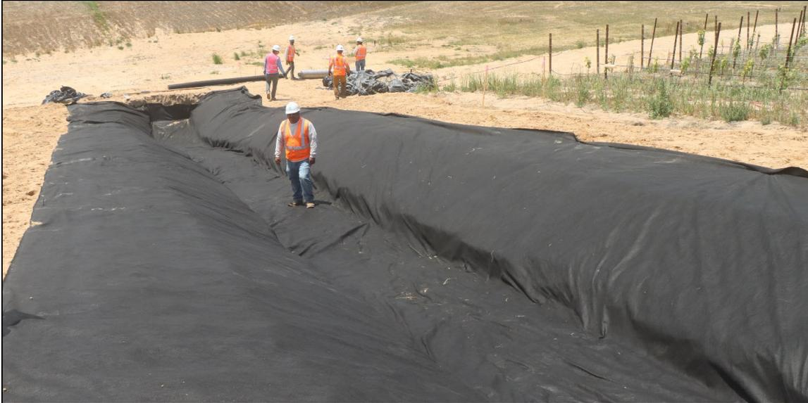
**Figure 1- Geotextile placement in excavation**
