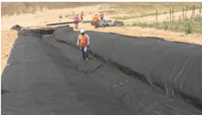
Figure 1: Geotextile placement in excavation
