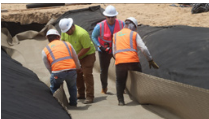
Figure 2: PROPEX Landlok HPTRM placement in bottom of excavation
