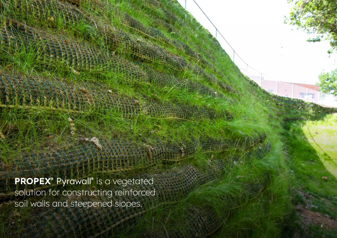
The system consists of PROPEX® Pyramat® 75 High Performance Turf Reinforcement Mat (HPTRM) and fiber-composite internal bracing. Featuring flexible setback and alignment, PROPEX Pyrawall can be customized to unique site conditions.
