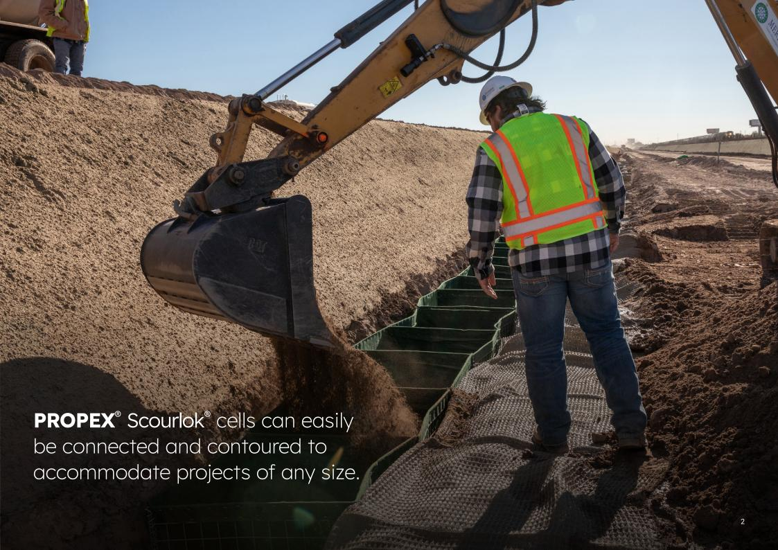
PROPEX Scourlok is a robust engineered bank stabilization system designed to resist extreme hydraulic stresses and protect shorelines while promoting vegetation.
