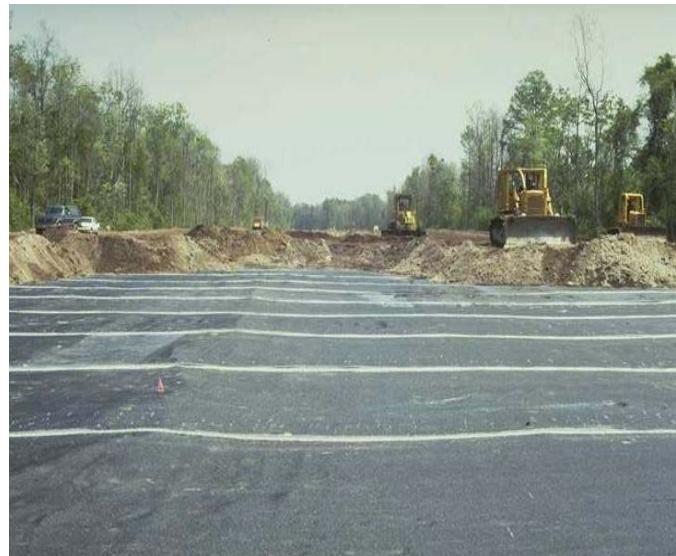
Figure 1. Seamed Geotextile Panel
