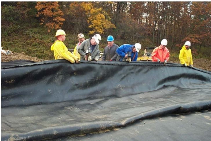
Figure 3. Field Sewing with hand-held machine hand-held machine.
