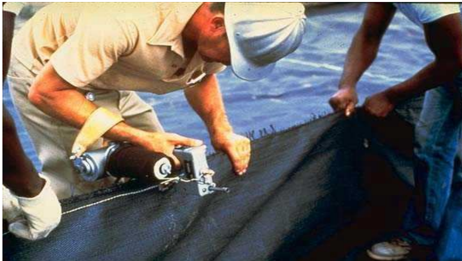
Figure 3. Field Sewing with hand-held machine
