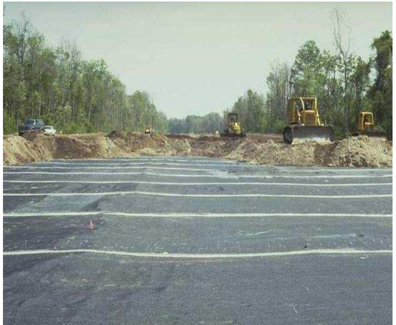
Figure 1. Seamed Geotextile Panel
