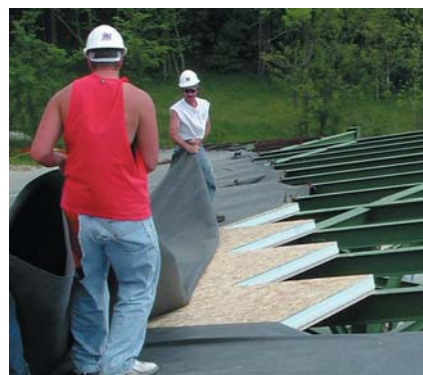
◀ Tectum III project installation.
