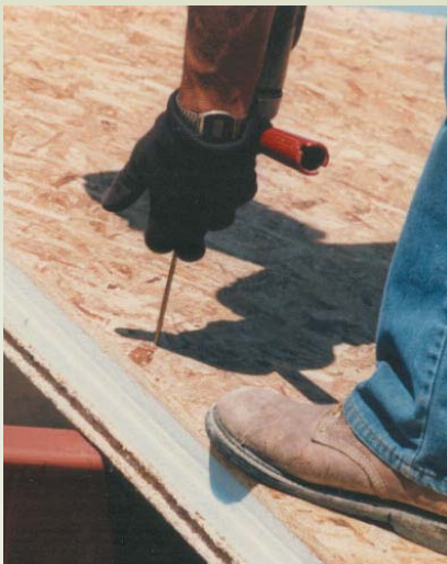
Tectum E installed over steel. ▲
