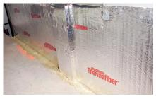
Tape over all Thermafiber<sup>®</sup> Spiral Anchors to restore vapor barrier with Thermafiber<sup>®</sup> Aluminum Foil or FSK tape.
