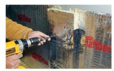
Mechanically attach the Thermafiber® Spiral Anchors using a Phillips head drill or electric screwdriver.
