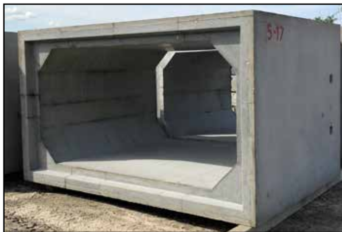
Finished Box Culvert
