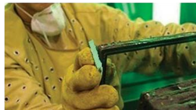
Eliminating cold joints and voids
