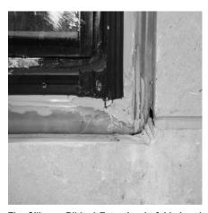
The Silicone Ribbed Extrusion is folded and sealed into the glazing pocket. Mechanical fasteners are used to hold the folded corner and are sealed over with Spectrem 1 Silicone Sealant.
