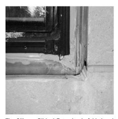
The Silicone Ribbed Extrusion is folded and sealed into the glazing pocket. Mechanical fasteners are used to hold the folded corner and are sealed over with Spectrem 1 Silicone Sealant.
