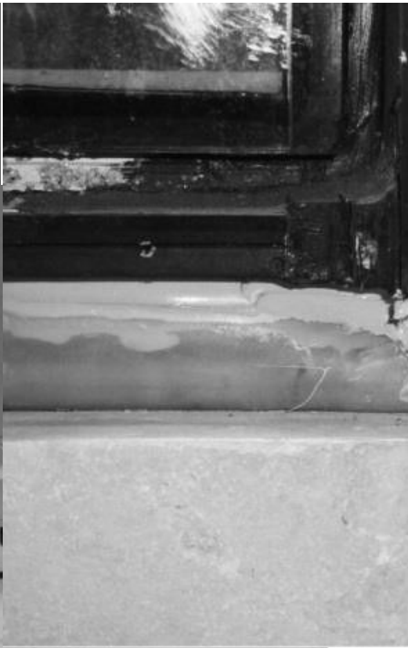
The Silicone Ribbed Extrusion is folded and sealed into the glazing pocket. Mechanical fasteners are used to hold the folded corner and are sealed over with Spectrem 1 Silicone Sealant.
