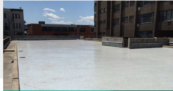
Completed System Prior to Asphalt Topping
