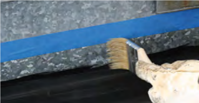
Prime all metal surfaces with M-Prime.
