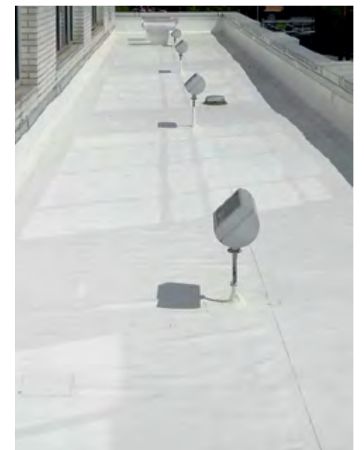
White single ply roof, cleaned and ready to be coated with AlphaGuard.
