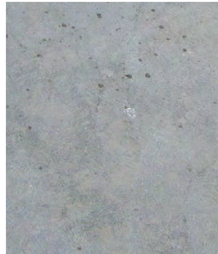
Properly prepared concrete substrate
