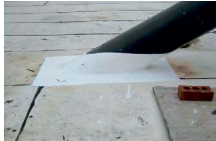
Penetrations on MB roof systems can be flashed with AlphaGuard as well.
