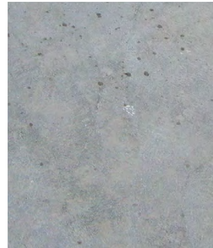
Properly prepared concrete substrate
