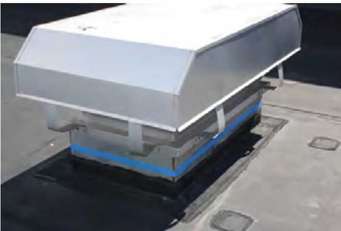
Tape all edges to provide a straight line for all flashing details.
