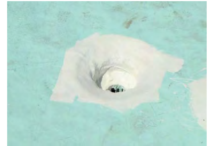
For concrete and insulated systems, extend AlphaGuard into the drain bowl. Ensure that the drain bowl is prepared per requirements.
