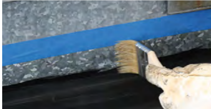
Prime all metal surfaces with M-Prime.
