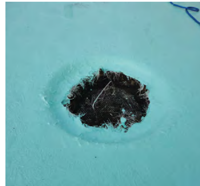
When flashing a drain, AlphaGuard will conform to the drain bowl, eliminating areas where water can penetrate.
