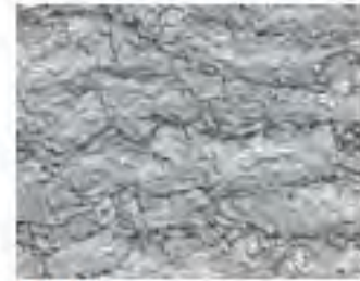
CSP 9 (Heavy Scarification)
