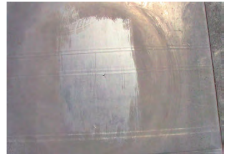
Holes and tears in membranes must be repaired before AlphaGuard is applied.
