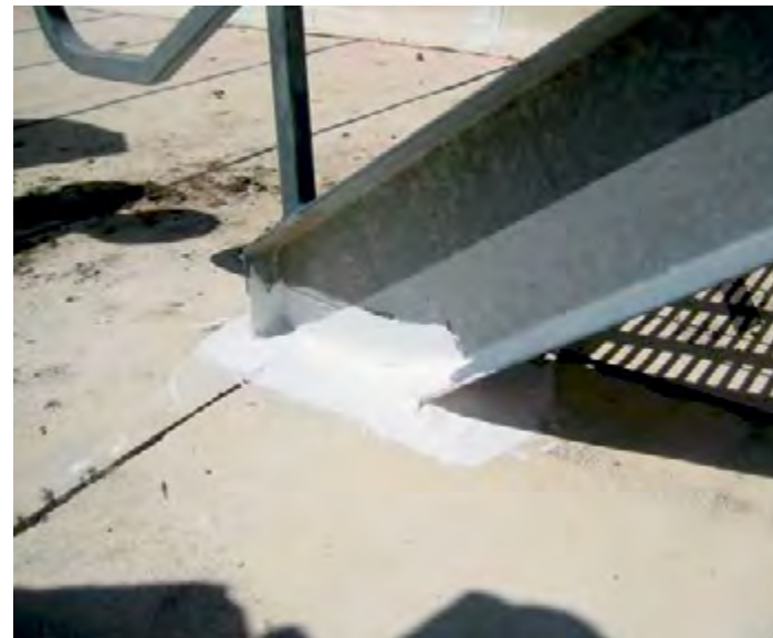
Penetrations that previously needed pitch pockets are flashed with AlphaGuard. This eliminates possible points of water infiltration.
