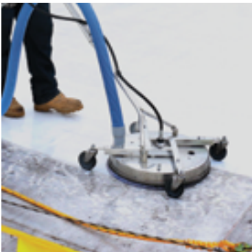
Step 1: Clean with RoofTec™
