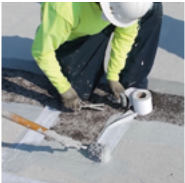
Step 2: Detail with Geogard Seam Sealer
