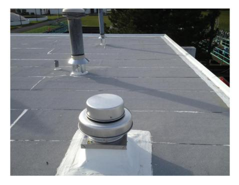
**Surfacing:** Multi-ply asphalt flashings require the application of a reflective coating. Two coats are recommended for best coverage.
