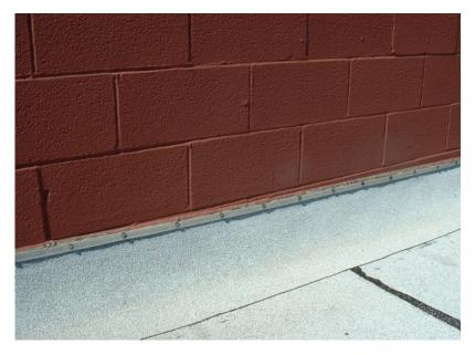
Base flashings shall extend onto the roof a minimum of 6" beyond the toe of the cant and a minimum 8" above the surface of the roof.
