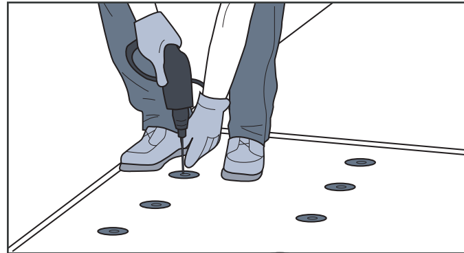
STEP 1 Insulation is fastened to the deck
