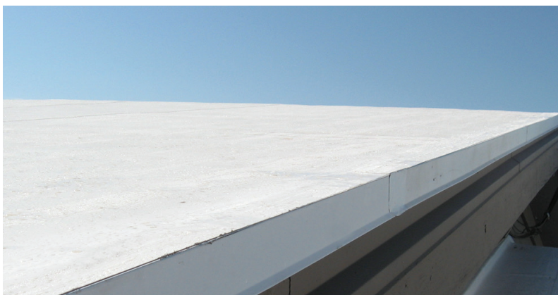
STEP 3 Seams are welded
