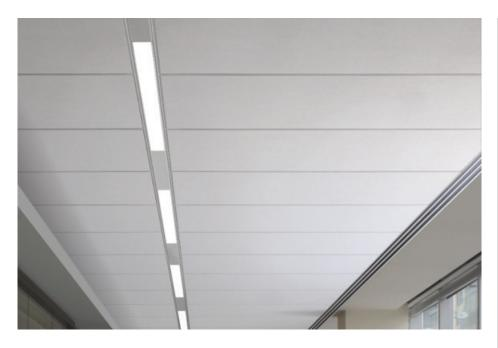
An innovative suspension system from USG, designed to accentuate design flexibility and product compatibility. A proprietary cap lance allows for extensive color and finish options delivering design freedom.
